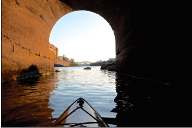
Looking downriver toward the Arch Bridge from the shadowy depths of the tailrace beneath a grinder room.
