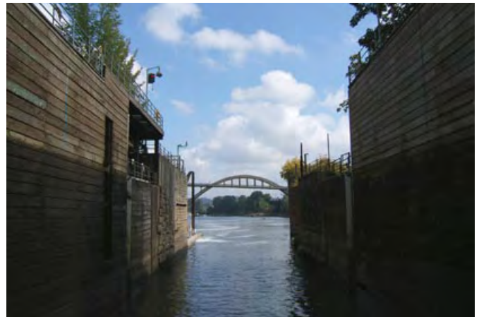
Lower entrance to 135-year-old Willamette Falls multiple-chambered navigation lock and canal.
