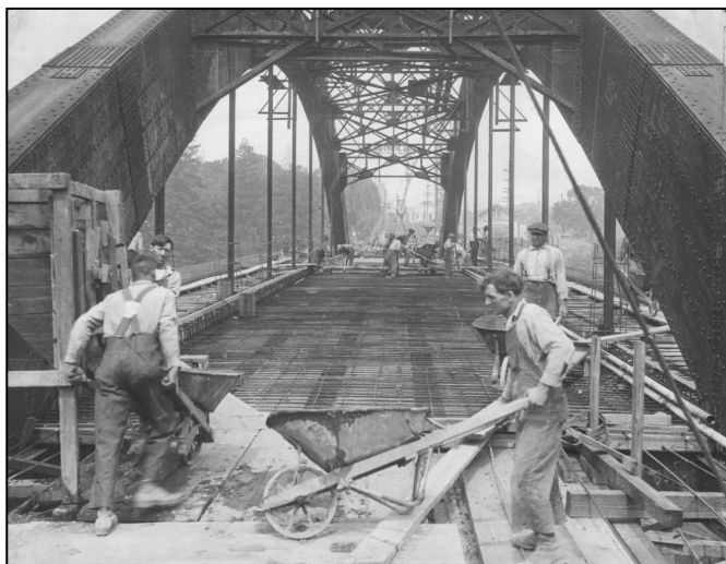
The back-breaking work of delivering concrete by hand formed the bridge's driving surface.
