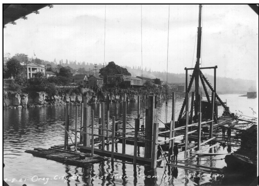
Framework for the building of the west side cofferdam. —Sept. 8, 1921
