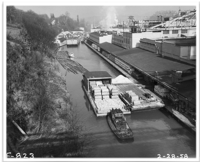
Built long before the advent of poured concrete construction, the lock walls were formed with basalt blocks quarried from the Carver area along the Clackamas River. They were hauled onsite by Chinese laborers and then hand-carved by European stonemasons. A testament to their craftsmanship, these walls have remained water tight for over 147 years!
