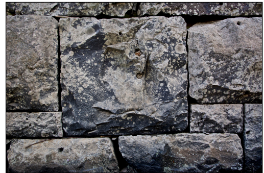
Built long before the advent of poured concrete construction, the lock walls were formed with basalt blocks quarried from the Carver area along the Clackamas River. They were hauled onsite by Chinese laborers and then hand-carved by European stonemasons. A testament to their craftsmanship, these walls have remained water tight for over 147 years!
