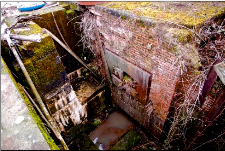
If one knows where to look on a Blue Heron mill tour, they would be surprised to see the face of an old boiler that remains on PGE’s dam. The brick structure sits directly next to the upper side of the dam and was part of Hawley Paper’s original Mill A.
